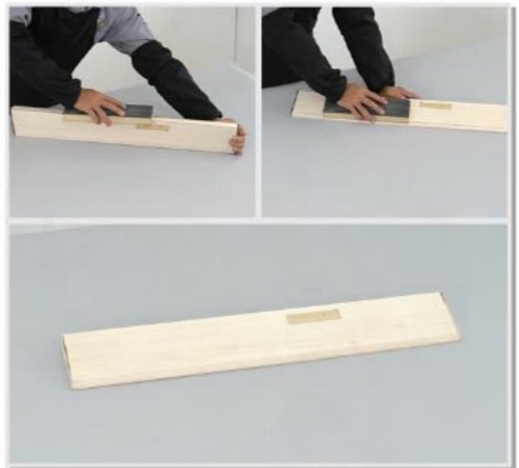
1.26 When glue is cured, remove rough edges with sand paper.
